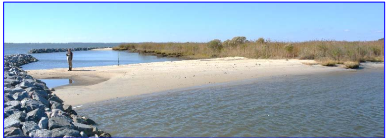
More heavy equipment placed sand behind the breakwater (above); the sand (below) will be planted in the Spring with two types of marsh grass, Spartina alterniflora and Spartina patens .
