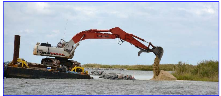
More heavy equipment placed sand behind the breakwater (above); the sand (below) will be planted in the Spring with two types of marsh grass, Spartina alterniflora and Spartina patens .
